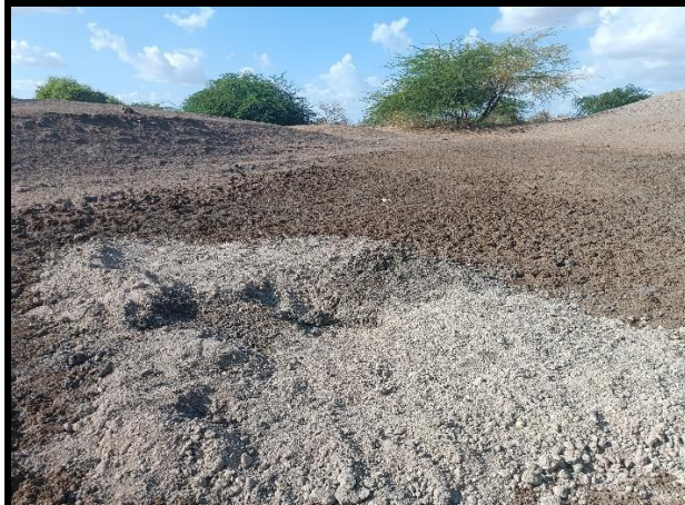
Proposed site identified for excavation the water pan showing a test pit for Soil Analysis for Water Retention Capacity.
